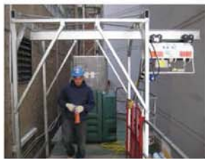
The Scaff-Trac and I-Beam Mounts adapt Beta Max Hoists to most continuous climbing scaffold and most climbing work platforms.
